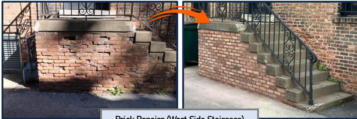
Brick Repairs (West Side Staircase)
